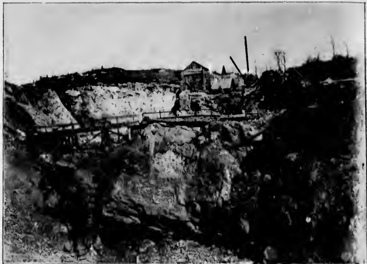
FIG. 86.—View of open-cut at south end of Mine Hill, Franklin Furnace, N. J., exposing the sycline of ore. From a photograph by J. F. Kemp, February 24, 1899.
